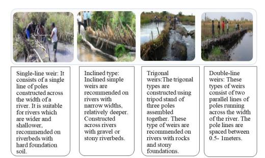
Fig. 2 Characterization of simple weir types and constructions methods
